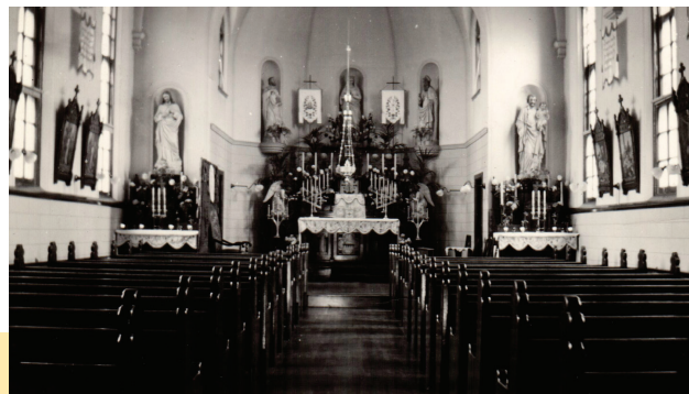
Historic View of Mullen Home's Chapel from the 1930's. The Chapel was recently remodeled, in 2018. This view highlights what Mullen Home's chapel originally looked like.
